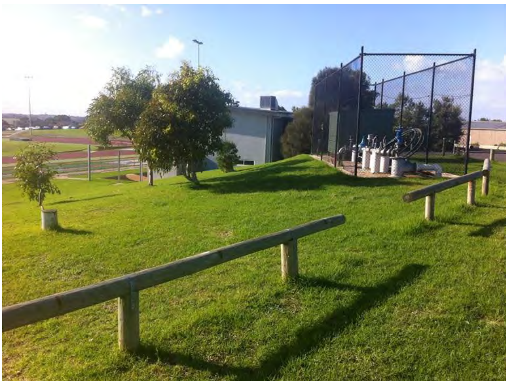
Figure 3.5 Stormwater filtering and aquifer injection system at Brauer College
